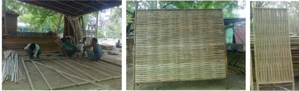
(a) Making of 2133 X 2743 mm 2 and 609 X 1828 mm 2 wall panel
