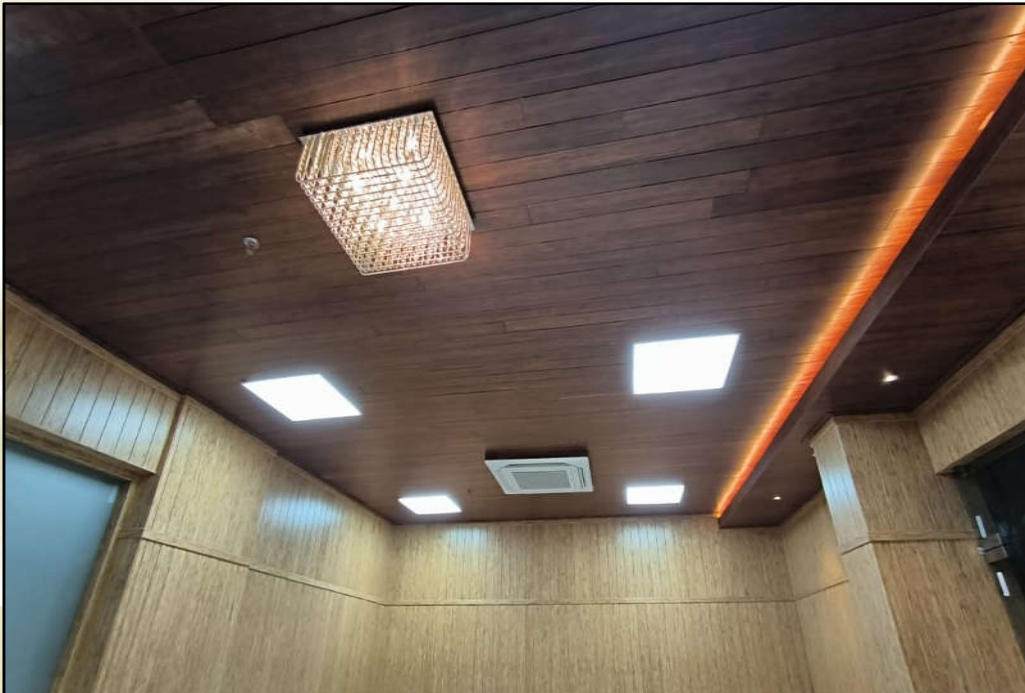
Bamboo Wood Ceiling installed @ Mohanbari Airport, Dibrugarh
